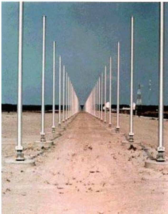
Figure 4.3-j : Monopole array of the ROTH system.
